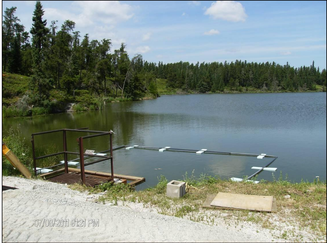
Figure 3.4 Photograph showing the pH adjustment system at the West Discharge.
