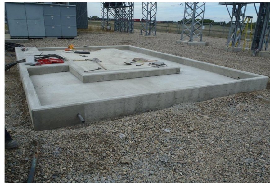
Photo 1: View of transformer foundation pre-installation
