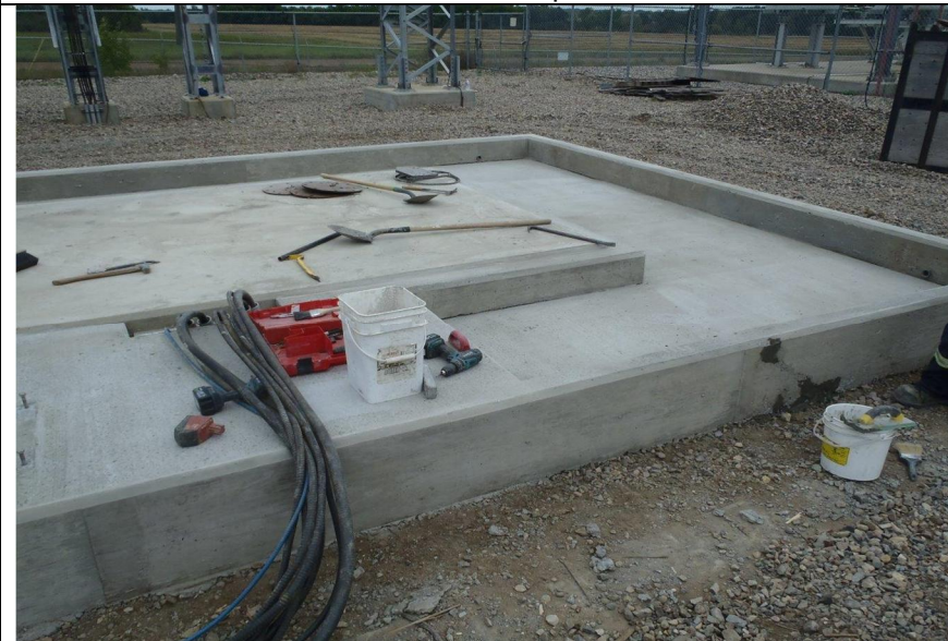
Photo 3: View of transformer foundation pre-installation
