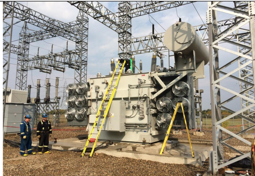
Photo 4: View of transformer during installation
