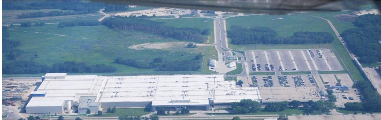
Boeing Canada Operations Ltd. Boeing Winnipeg Murray Park Facility – Aerial Photograph
