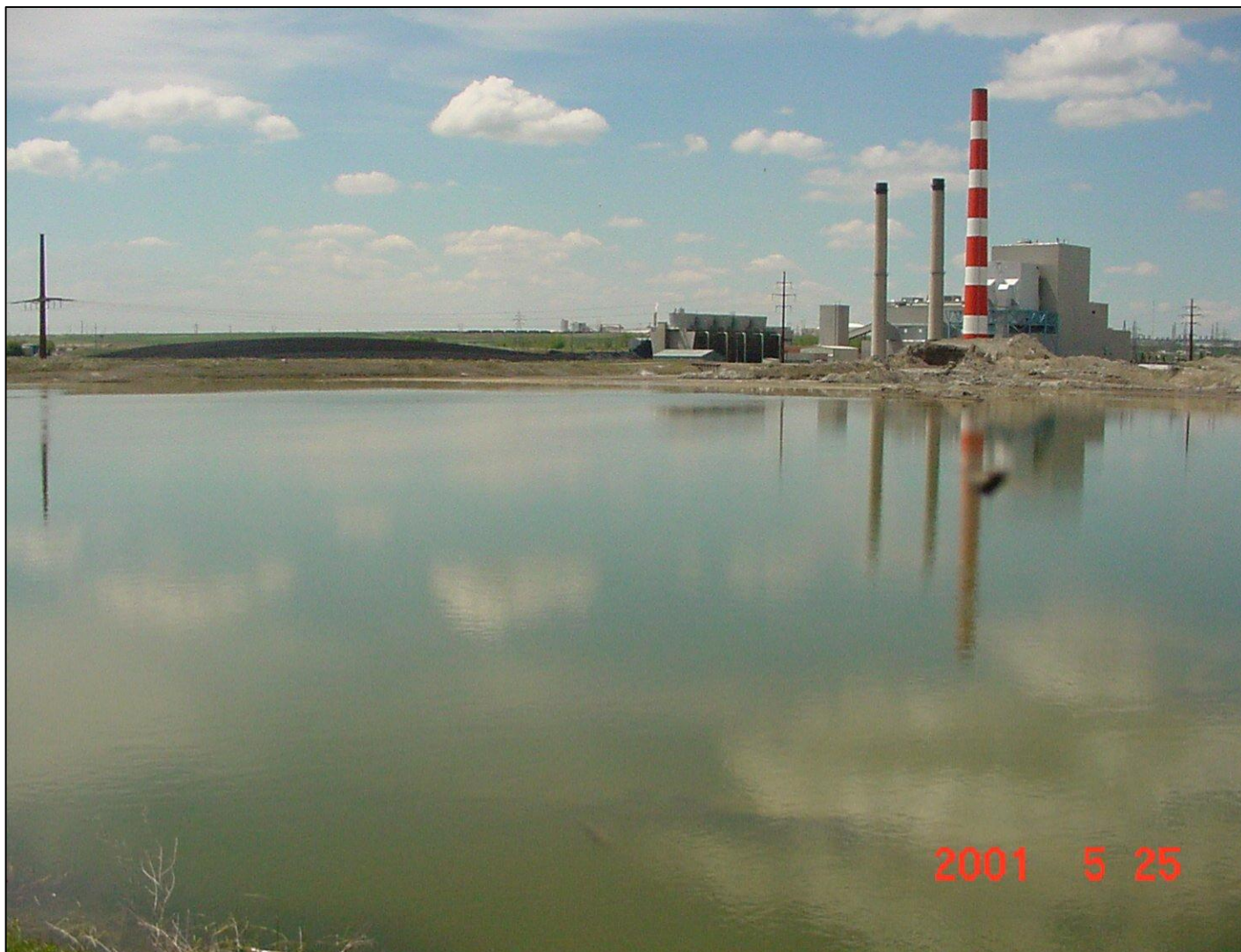
ASH LAGOON SETTLING POND
