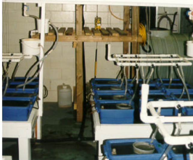
Water distribution tower with the river water and ammonia distribution chambers Figure 3-7
