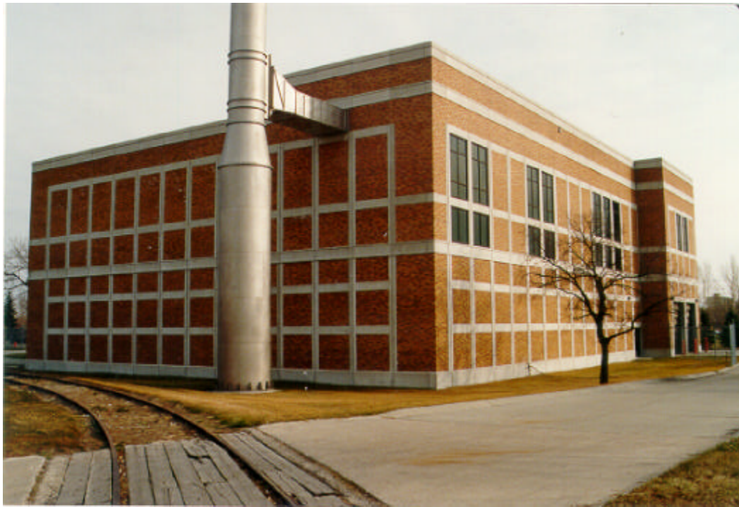
Location of the continuous flow toxicity lab at the dewatering building, City of Winnipeg North End Water Pollution Control Center
