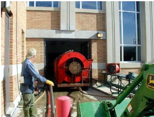
Motor Being Removed from Main Building
