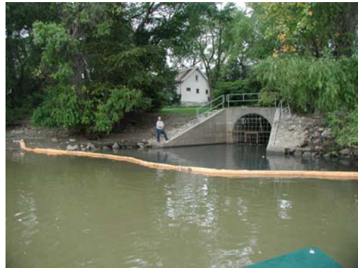
Boom Placed in the Red River to Catch Floating Debris at the Jefferson Outfall
