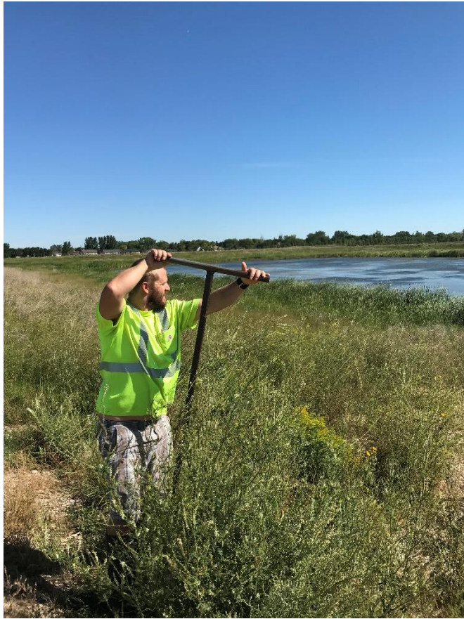
Figure 12. Town of Niverville employee Andrew Rempel opening connection between wetland and holding cell (August 10, 2020).
