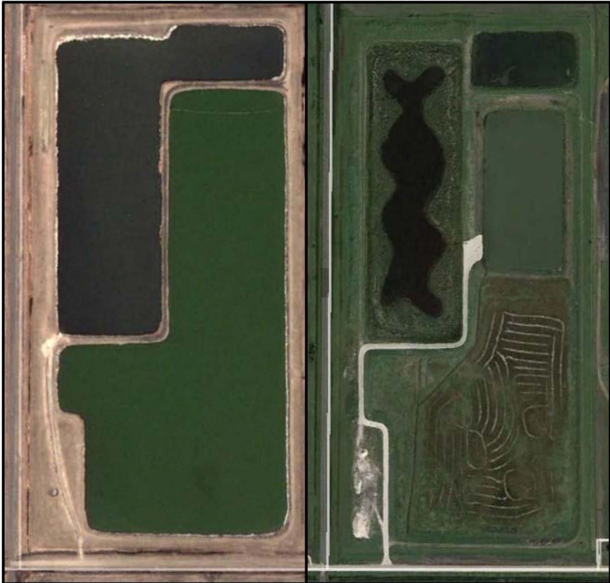
Figure 2. Niverville lagoon on SW 30-7-4 EPM during operation in 2002 (left; Image courtesy of Google Earth; Imagery date: May, 2002) and in 2016 after redesign for the Niverville Lagoon Bioremediation Project (right; Image courtesy of Google Earth; Imagery date: 2016).
