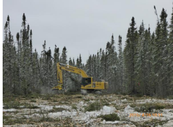
Photo 6 Transmission Line clearing using rotary blade on an excavator
