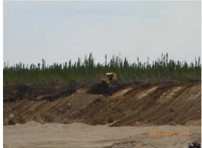
Photo 23 Spreading of stockpiled soils over borrow pit slopes.
