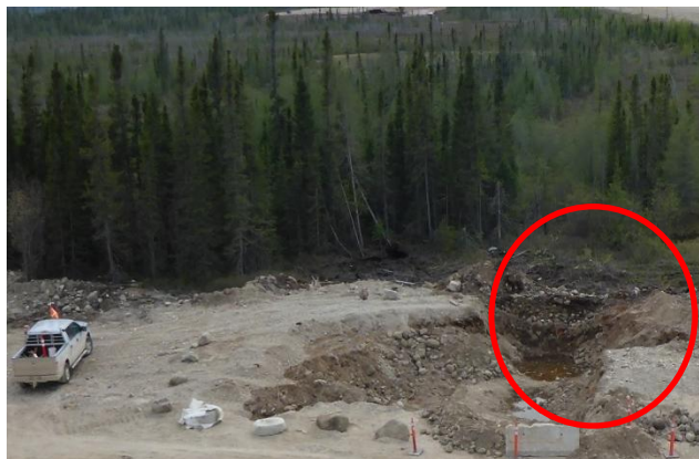
Photo 24 Excavation of Petroleum Fuel Storage Area at Keewatinohk
