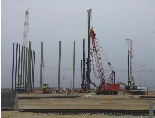
Photo 5 Installation of concrete piles for the Riel Converter Station
