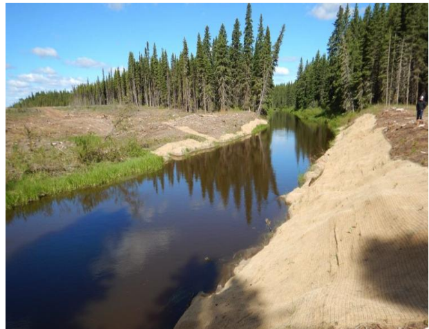
Photo 9 Erosion Control Blanket installed at Mitishito River crossing.
