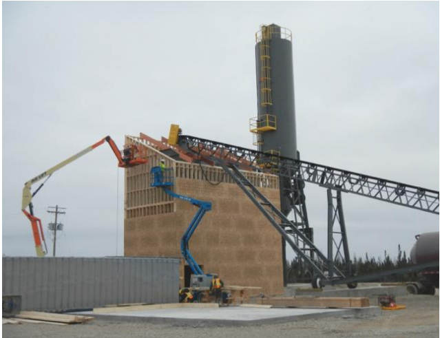
Photo 4 Installation of concrete batch plant at Keewatinohk
