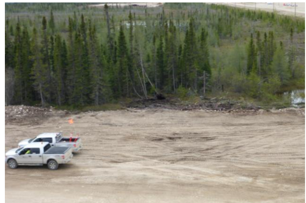
Photo 25 Completed Excavation of Petroleum Fuel Storage Area at Keewatinohk
