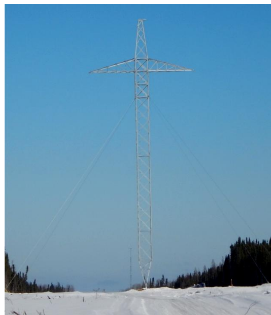
Photo 1 Newly erected tower on construction segment N2
