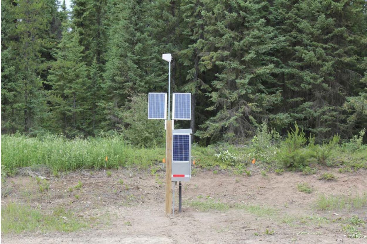
Figure 1 Traffic monitoring station
