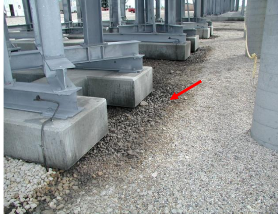
Photo 3: PHC (oil) staining on surface gravel
