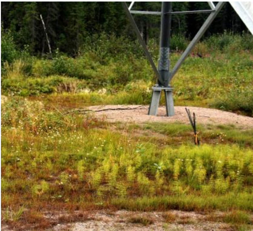
Photo 2. Photo of a transmission tower in a wetland under non-frozen ground conditions.
