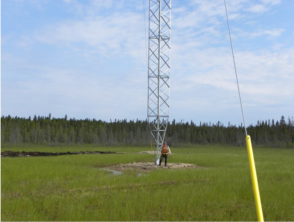
Photo 3. Photo of a transmission tower and guy wires in wetland in non-frozen ground conditions.
