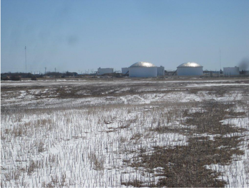
Photoplate 37 - View SE at second deflection pt on pipeline route in NW 20-09-28 WPM.
