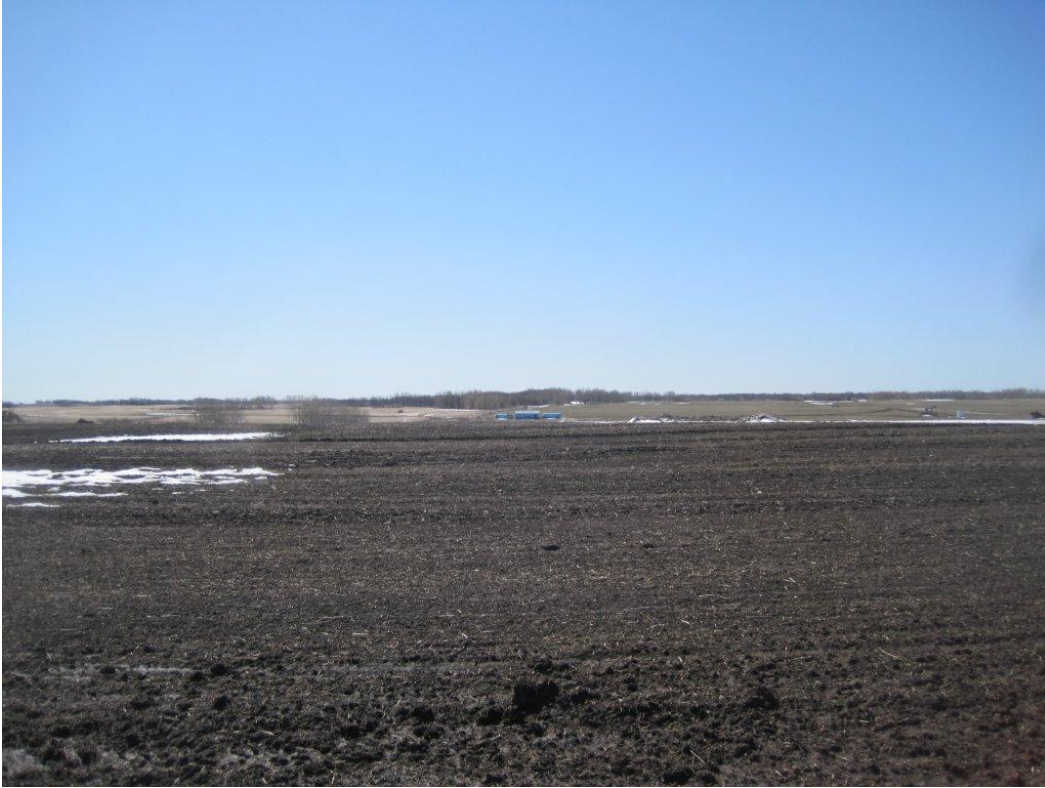
Photoplate 13 - View south on pipeline route in NE 07 at existing A/R to Battery 09-07-10-28 WPM.
