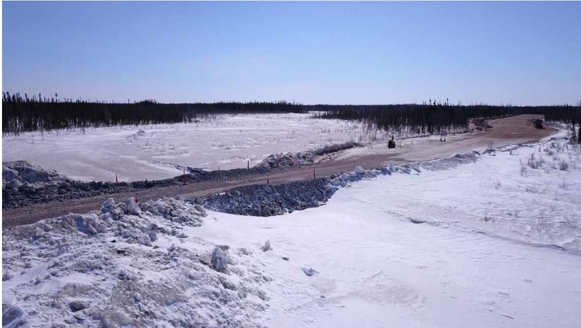
Photo 1. Temporary creek crossing on winter road to Ellis Esker, April 7, 2018
