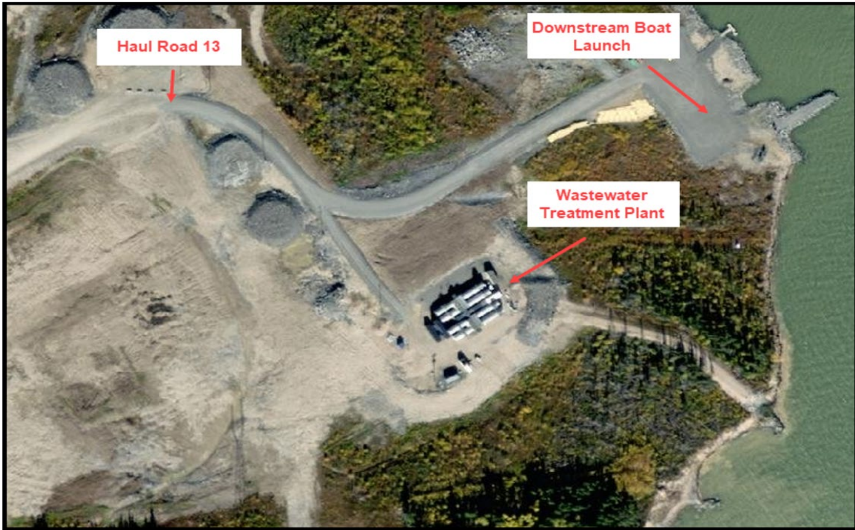
Photo 2. Keyyask Wastewater Treatment Plant infrastructure.
