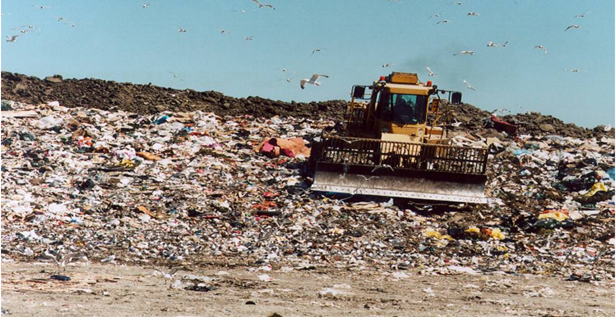
Photo 2: Typical working face and compaction equipment
