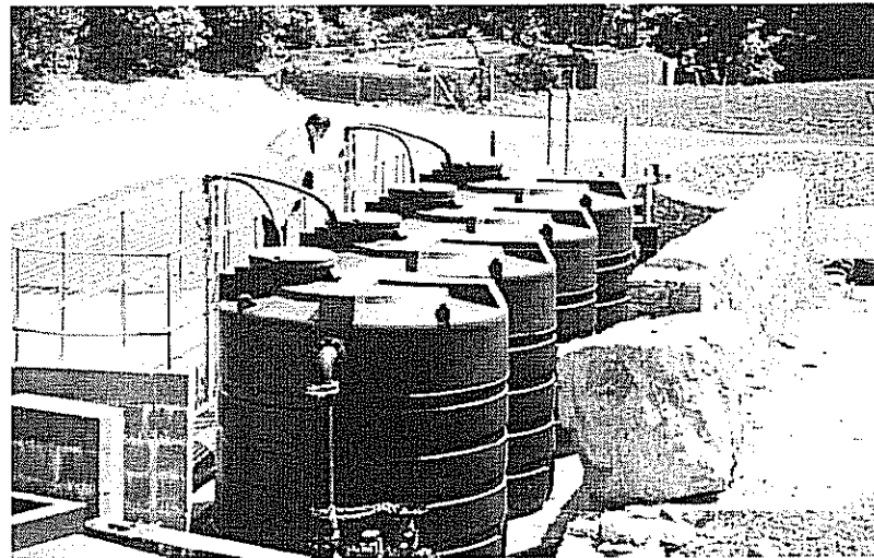
Figure 4.2: Typical Aeration Tank Installation
