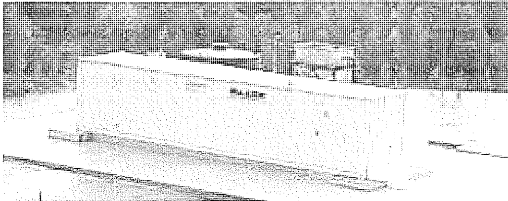
Figure 2.3: Typical Container Mounted RO Modular Plant
