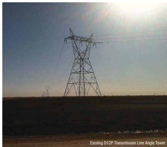
Existing D12P Transmission Line Angle Tower
