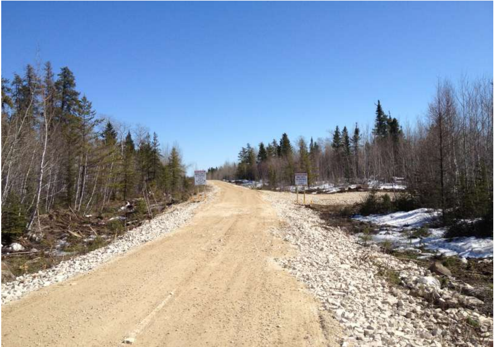
Access Road – Looking East
