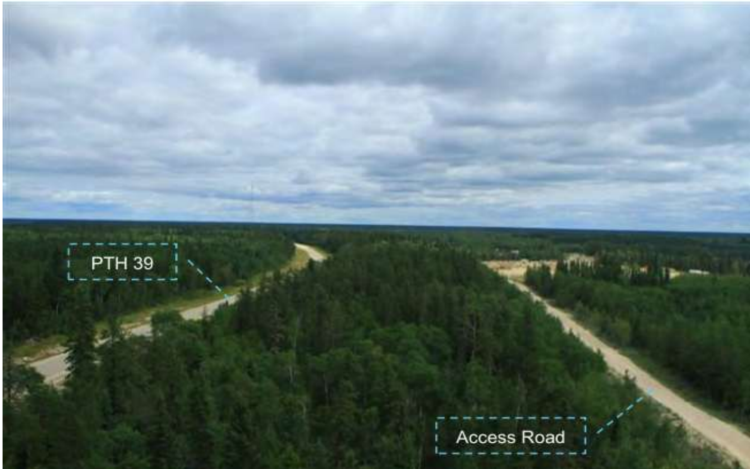
Reed AEP Site and Access Road on right, PTH 39 on left, looking east (August 2012)
