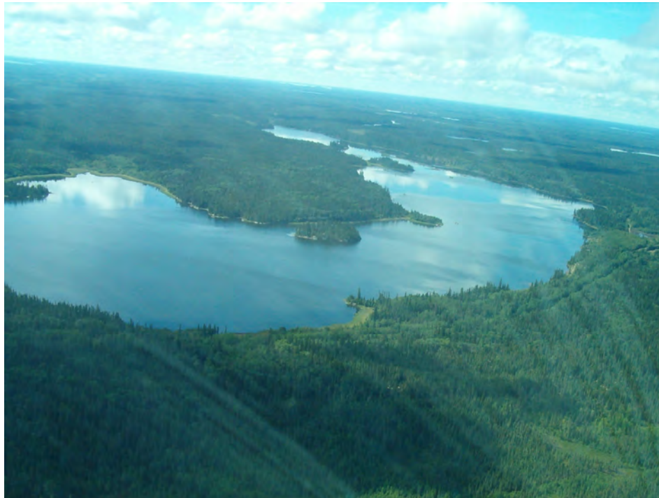
Photo 6: Anderson Tailings Impoundment Area (TIA)
