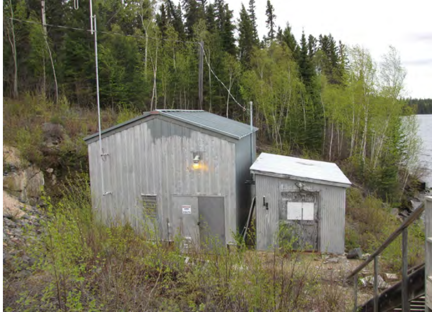
Photo 5: Snow Lake Pumphouse
