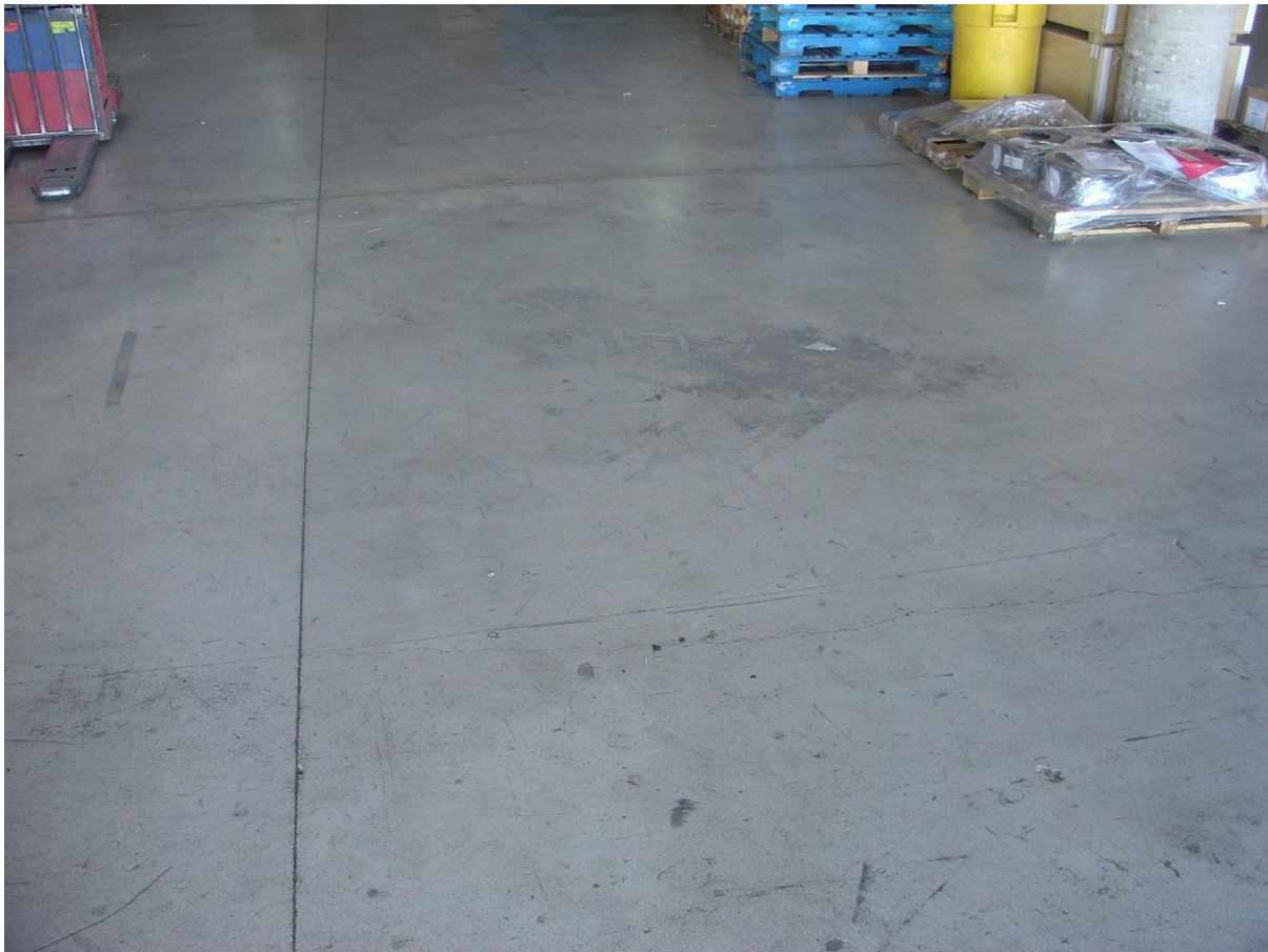
Figure 4: Floor in area where batteries were wrapped on pallets. Staining visible on floor is not related to battery operation.
