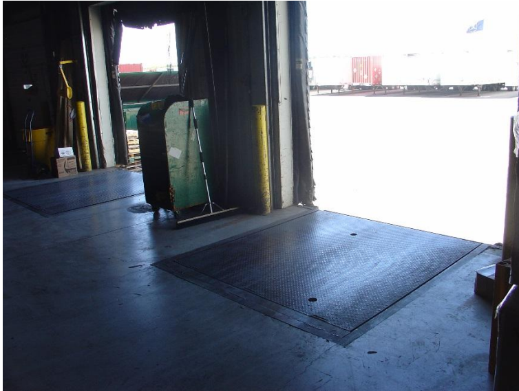
Figure 3: Loading and unloading dock areas that were used for battery transfer.
