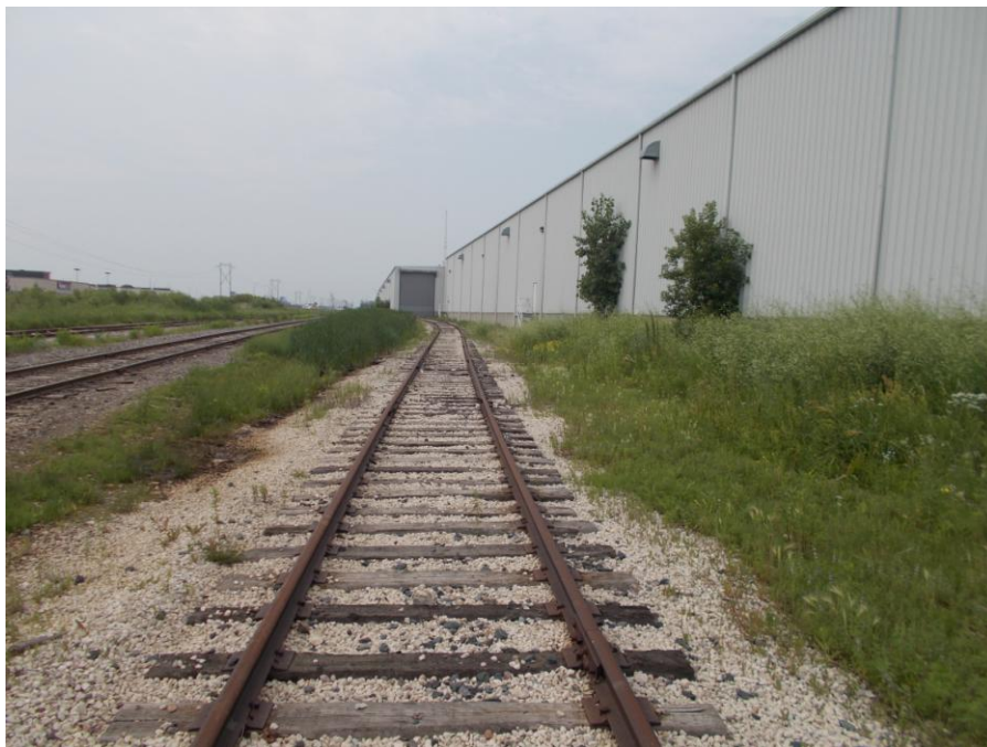
PHOTOGRAPH 4: Looking south showing the rail spur leading into the Site building.
