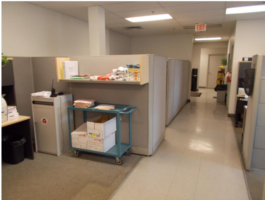
PHOTOGRAPH 5: Showing typical interior building materials observed in the office space located in the northwest corner of the Site building.
