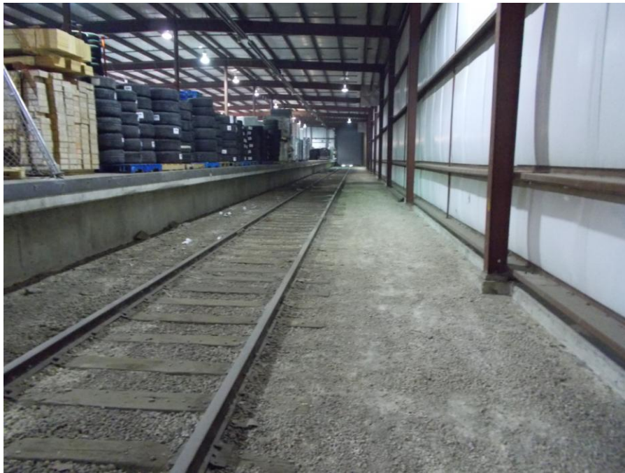
PHOTOGRAPH 10: Showing the rail line located within the cross dock area of the Site building.
