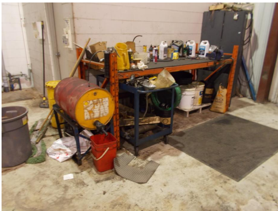
PHOTOGRAPH 12: Showing the chemical storage area for forklift maintenance equipment and supplies in the maintenance room.
