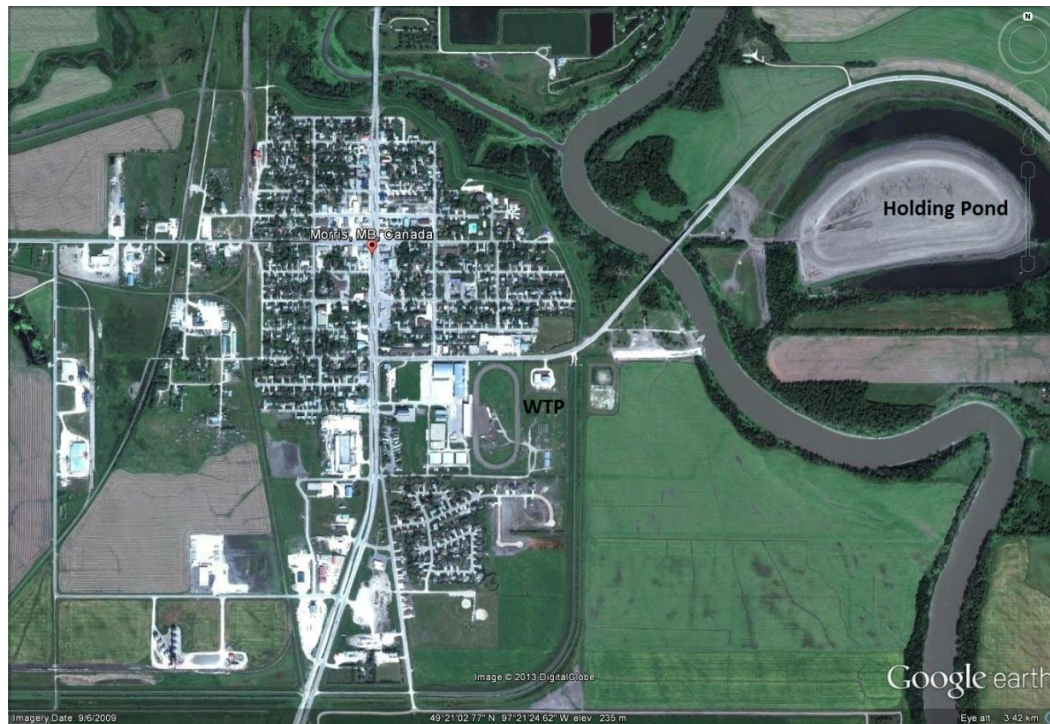
FIGURE 2.1- LOCATION OF MORRIS REGIONAL WTP AND HOLDING POND
