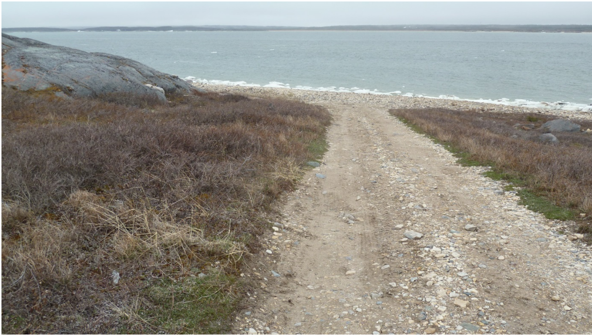
Photo 5 – Access road to Churchill River.
