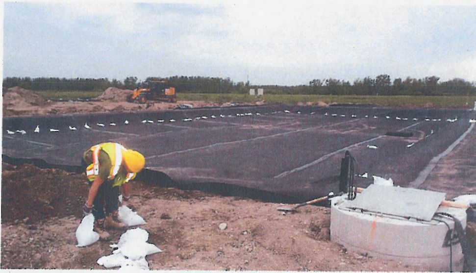
13. Cell #1 Placement and Wedge Welding Complete
