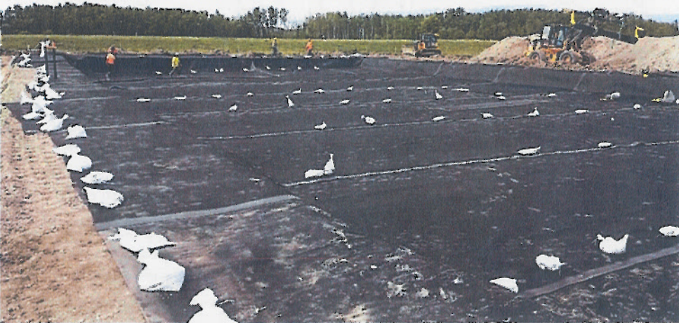
3. Cell #2 Placement Complete
