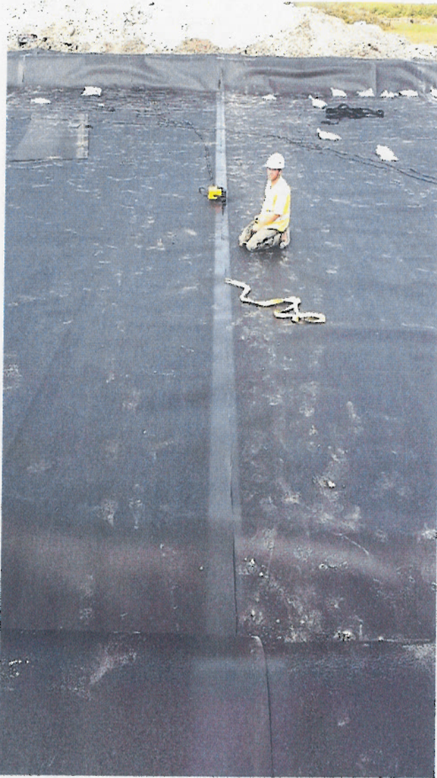
7. Welding in Cell #2- white line indicates 125 mm (5") overlap
