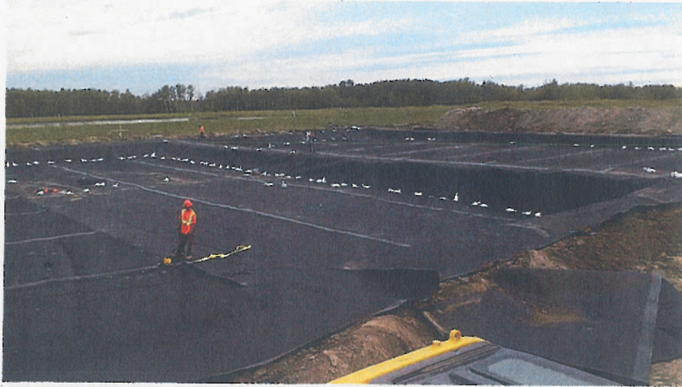
12. View of both cells – final butt seam welding
