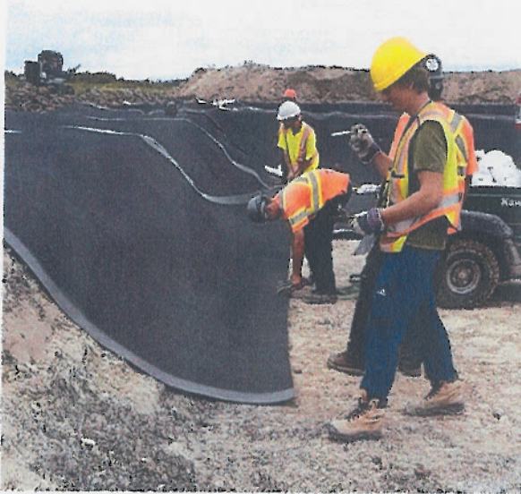
9. Clamp detail – ½” diameter bars on clamp prevent marring of liner
