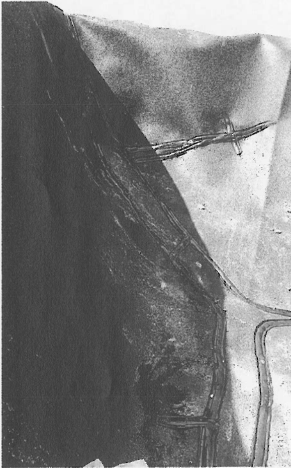
17. Extrusion welding on complex sloped corner
