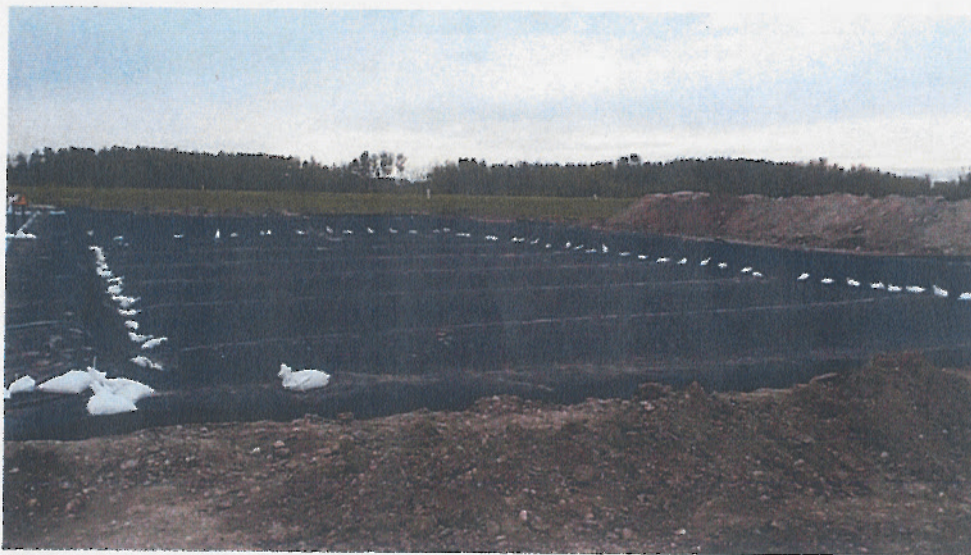
14. Cell #2 Placement and Wedge Welding Complete
