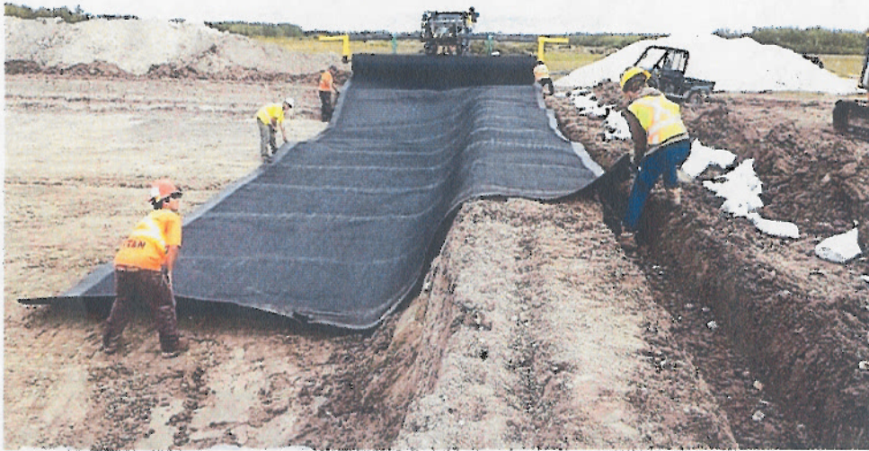
1. Placing First Roll in Cell #2 by hand
