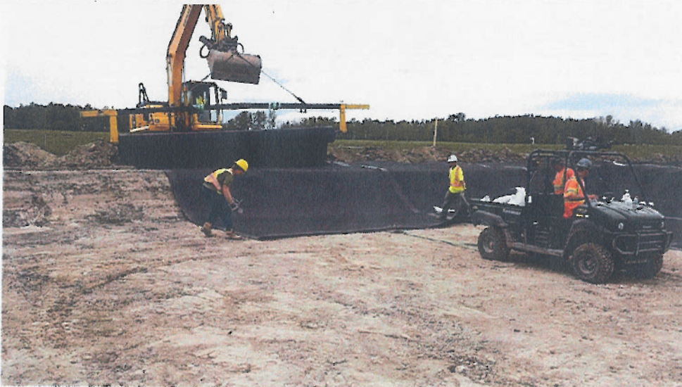
8. Machine assisted placement in Cell #1
