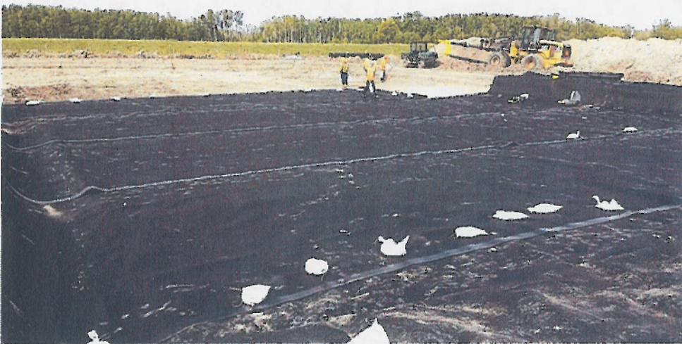
2. Part way through placement in Cell #2
