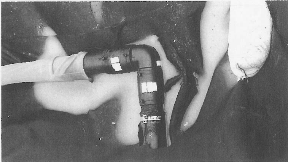
18. Finished Pipe Penetration in Cell #2 (with geo-cushion and drain pipe)
