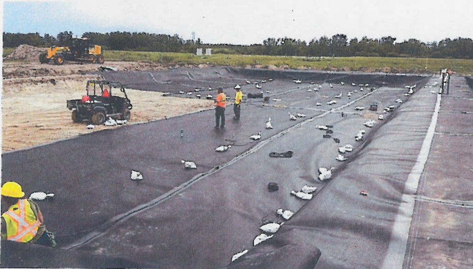
10. Partially Completed Cell #1
