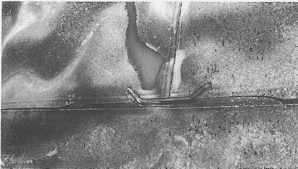
16. T- weld reinforcement detail along butt seams
