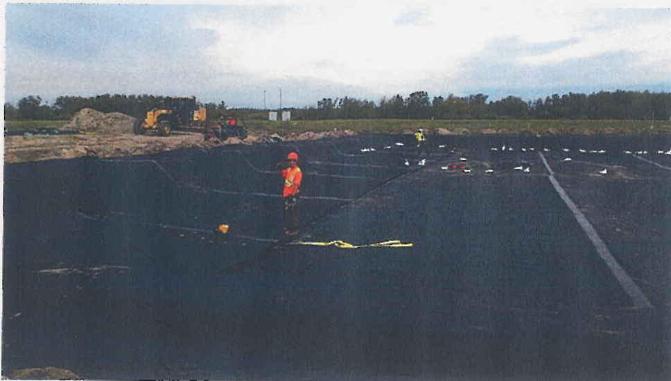
11. Completed placement in Cell #1
