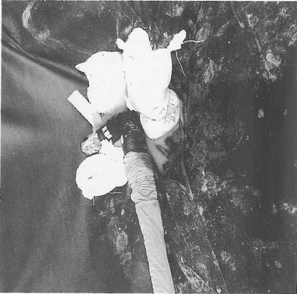
19. Finished Pipe Penetration in Cell #1 – with geo-cushion and drain pipe
