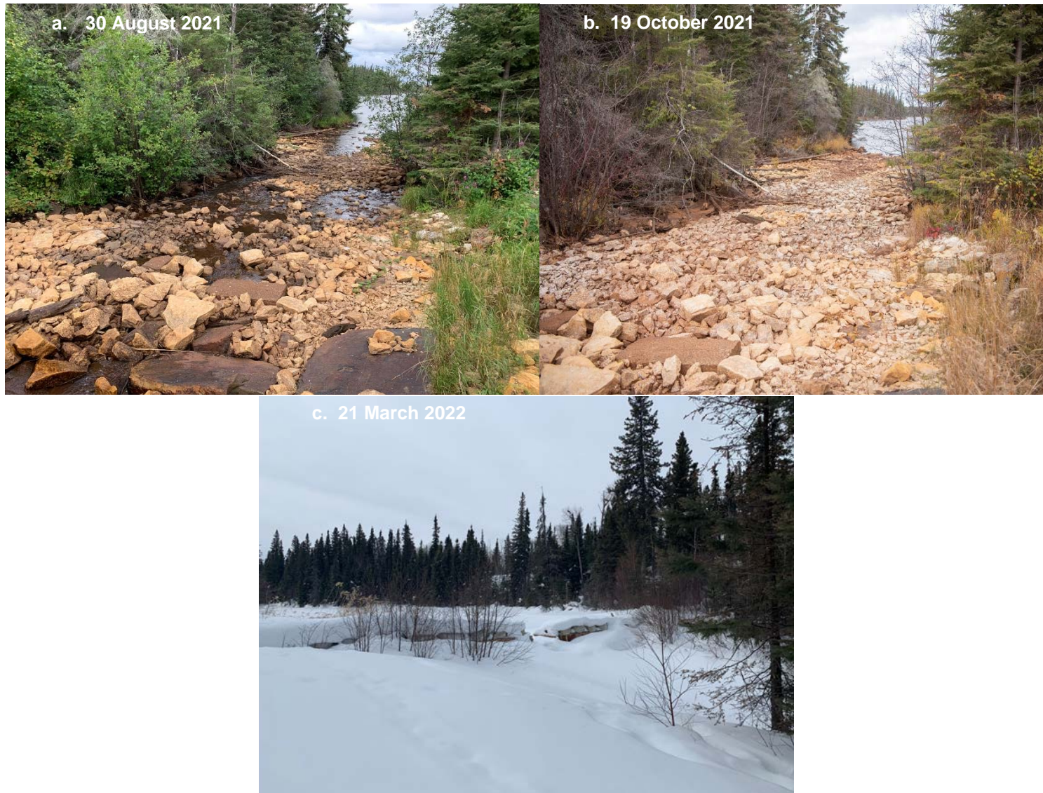
Figure 7. Camp Lake Discharge Spillway. a. 30 August 2021. b. 19 October 2021. c. 21 March 2022.
