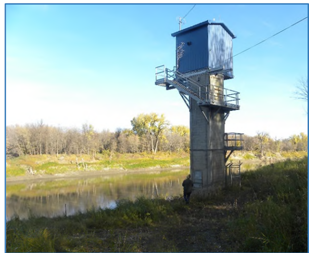
Water Survey of Canada water level and flow monitoring station.
