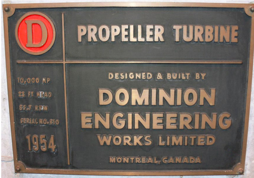
Figure 14 Unit No. 8 Nameplate Original
