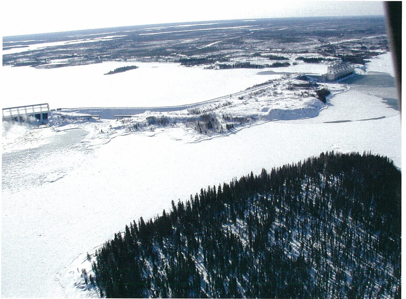
Photograph 1: Kelsey Generating Station Powerhouse and Spillway
